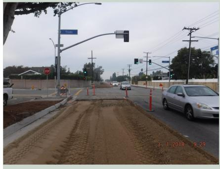
The traffic signal modification will be completed along with the asphalt concrete finish course on Main Street to prevent cutting into new pavement. Manholes, monitoring wells, survey monuments, and water valve assemblies will be adjusted to grade and traffic loops and striping will be replaced. Areas of raised or settled curb gutter and sidewalk will be replaced.
