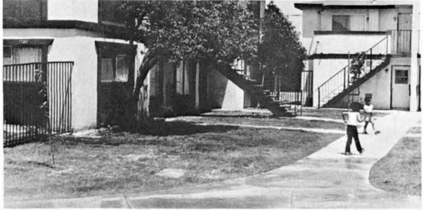
KOLEDO LANE —The new look of the Koledo Lane apartment complex. The much-needed improvements were done as a part of the city Housing/Rehabilitation loan program.
